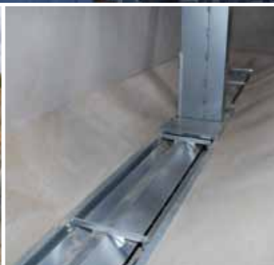
Chain elevator with side auger on both sides in grain pit.
