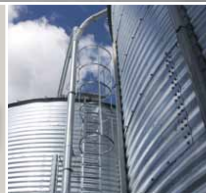
Pipe assembly for filling outdoor steel silos.
