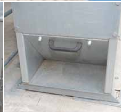
Access to elevator boot emptying.
